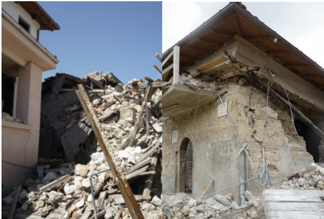
Figure 1. Completely failure (left) and partial failure (right) [3]
